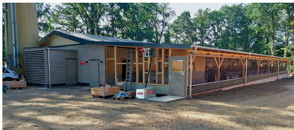
△ The 400-place fattening farm in Lower Saxony was converted into an animal welfare barn and the old building was extended to include an outdoor climate area and a manure/urine separation system
